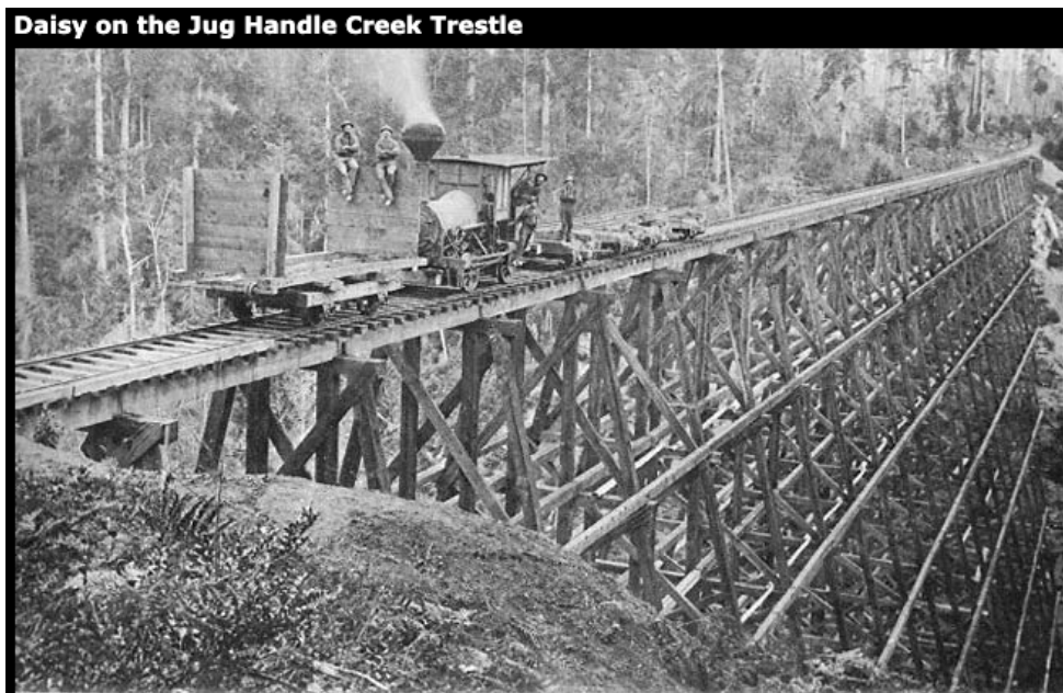
Figure 14: The world’s largest wooden trestle over Jughandle Creek, 1889. (see Maps 4 & 5)
